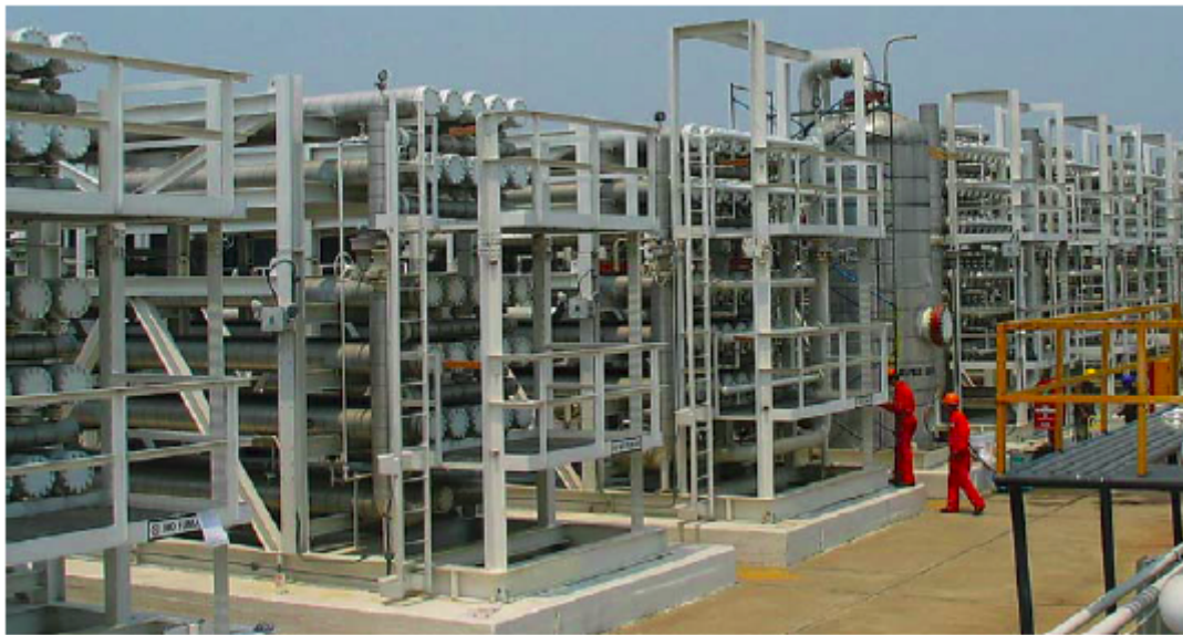
Figure 3 – Separex membrane skids installed at an EOR project in Latin America 6 .
