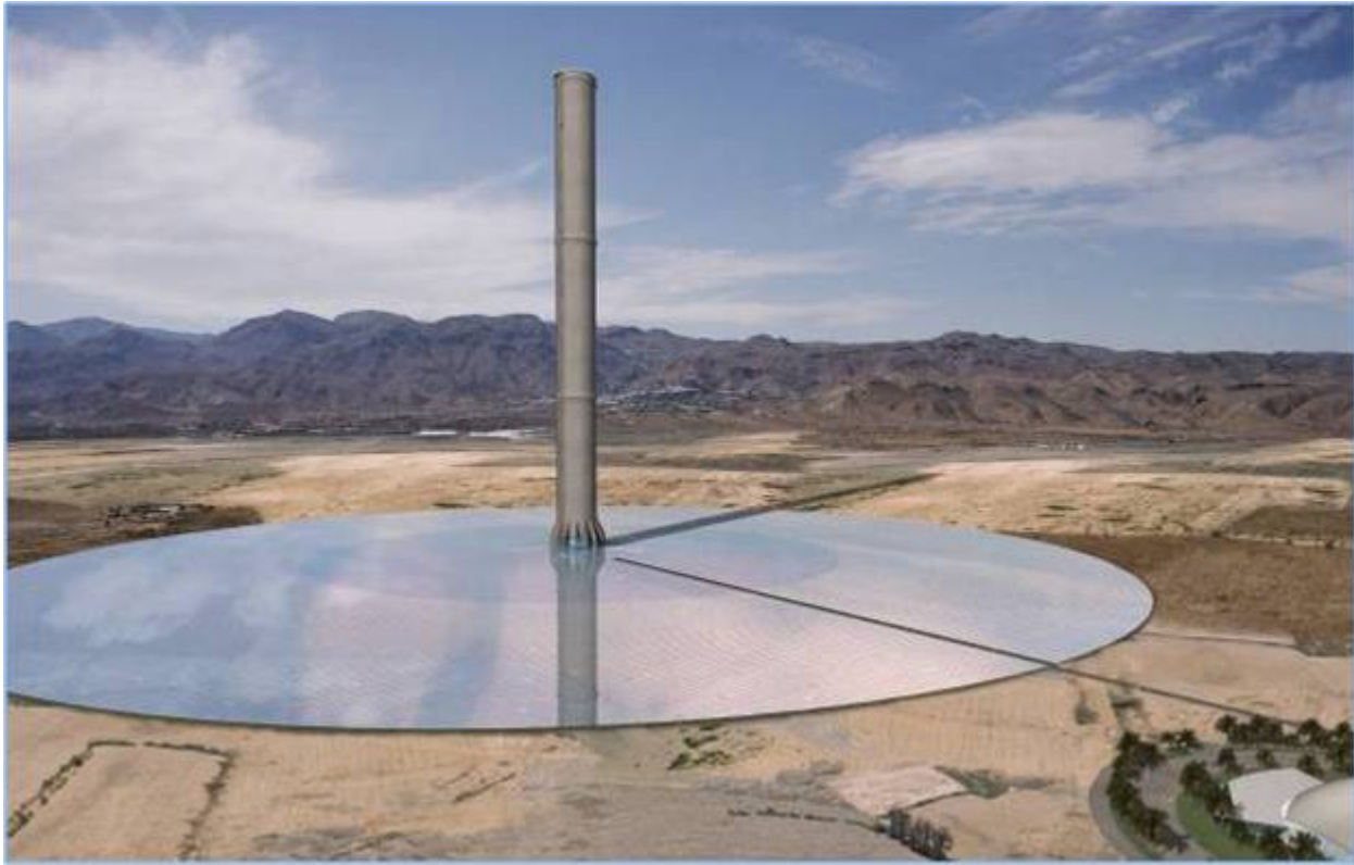
3D Rendering of 5 MW solar chimney power plant [8]
