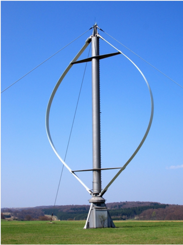
Fig. 4 – Darrieus turbine
