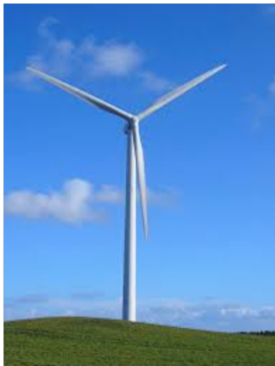
Fig.3 – Horizontal-axis wind turbine
