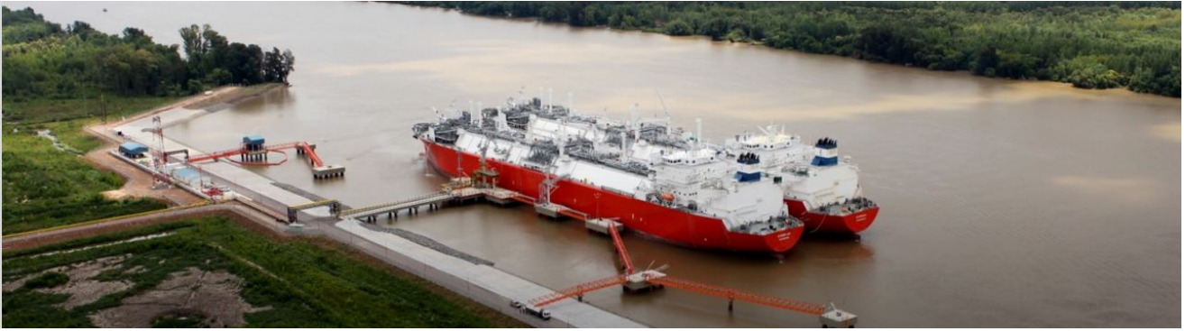
Fig. 4 – FSRU vessel for LNG transportation and regasification
