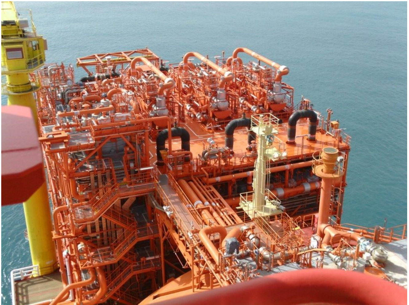
Open Rack Vaporizer Installation on FSRU
