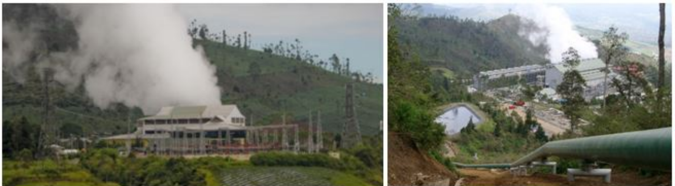
Fig.8 – Darajat Power Station, Indonesia
