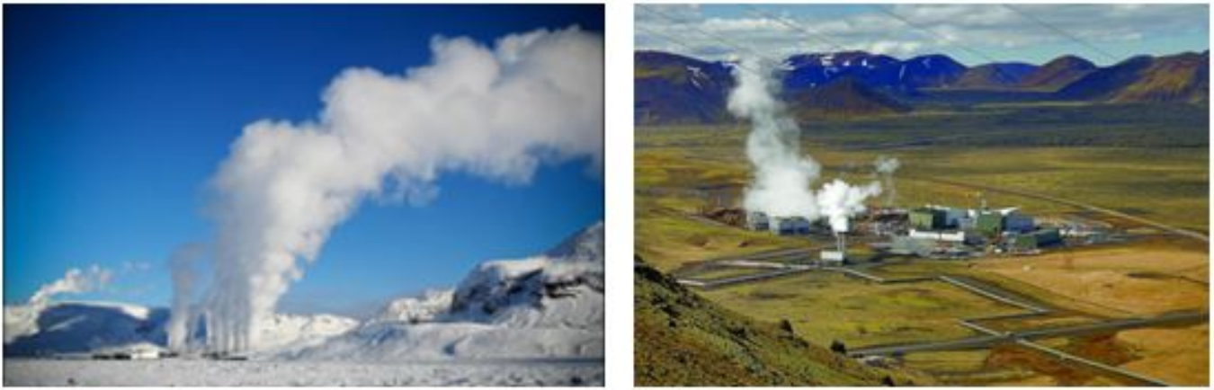
Fig.6 – Hellisheidi Geothermal Power Station, Iceland
