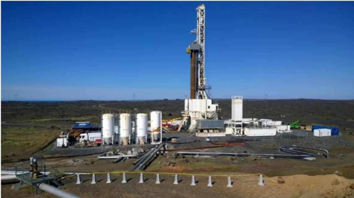
*Fig. 1 Geothermal Well at Iceland Deep Drilling Project – IDDP-2 well was completed at 4,659 meters depth searching for a supercritical steam zone*
