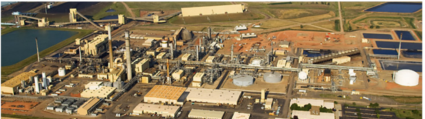
Great plains synfuels plant (GPSP) in Beulah
