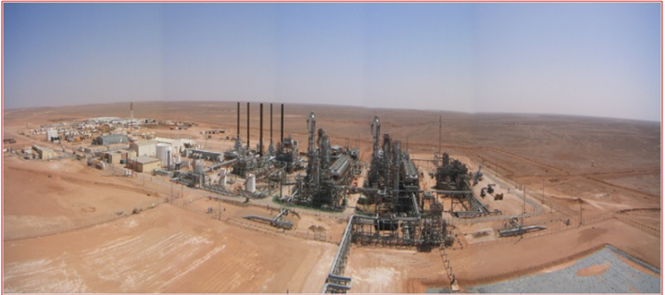
Fig. 4 – In Salah onshore industrial-scale CO 2 storage site
